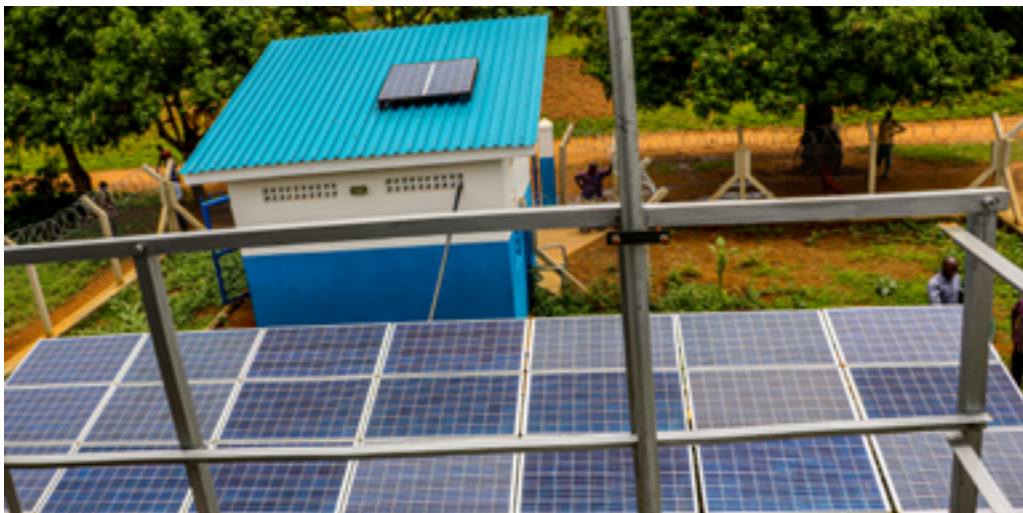
Figure 1: Typical Uganda WSSP Mini Solar-Powered Pumping Scheme
